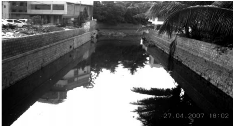
Plate 5.7: Remodelled storm water drain
