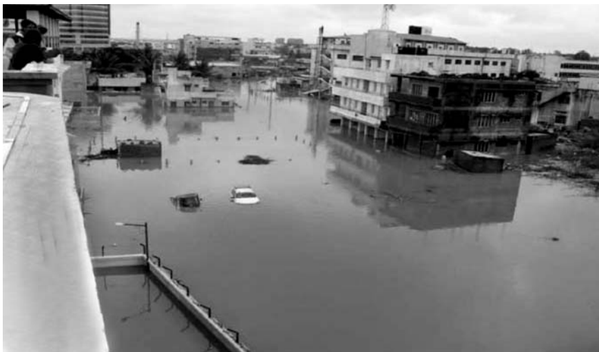
Plate 4.3: Flooding In Banashankari (Photo: Ranjini)
