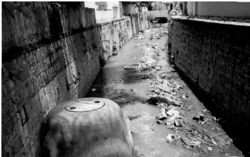
Plate 2.5: Sewer manhole and dumping of solid waste – reducing channel section (Source: BWSSB)
