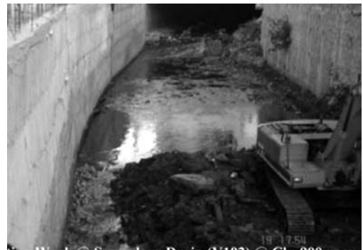
Plate 5.6: Construction of RCC box drain in Puttenahalli (Source: BMP)
