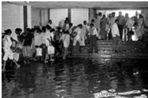
SUBWAY BETWEEN MAGESTIC AND RAILWAY STATION
