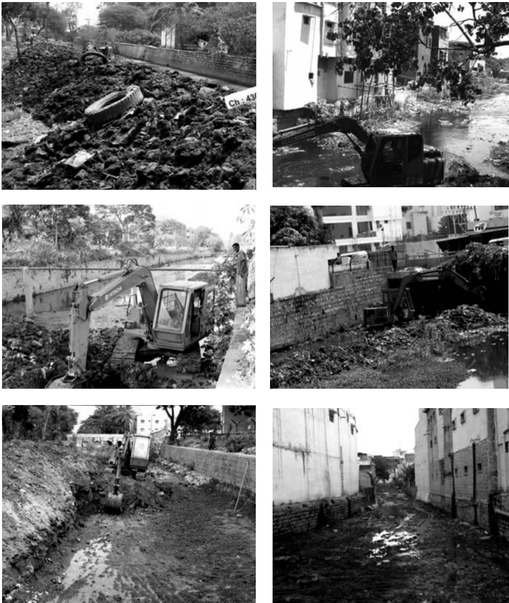
Plate 5.4: Desilting in Koramangala main valley, KH Road and Chalgatta valley
