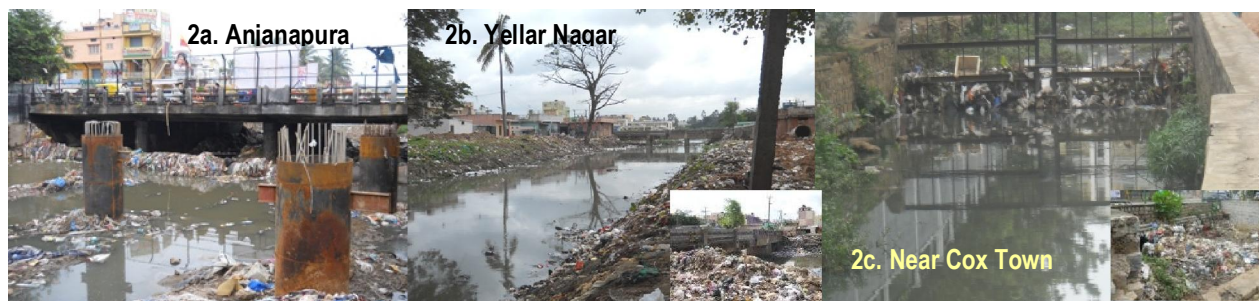
Figure 2: Details of the three study sites subject to urban flooding. Photo insets indicate the choked area while stagnant water in larger photo shows blockage of regular flow.
