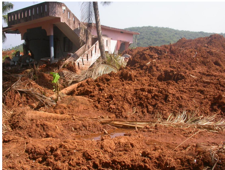
Figure 5: A house that was drifted and destroyed in the Kadwad-2 landslide
