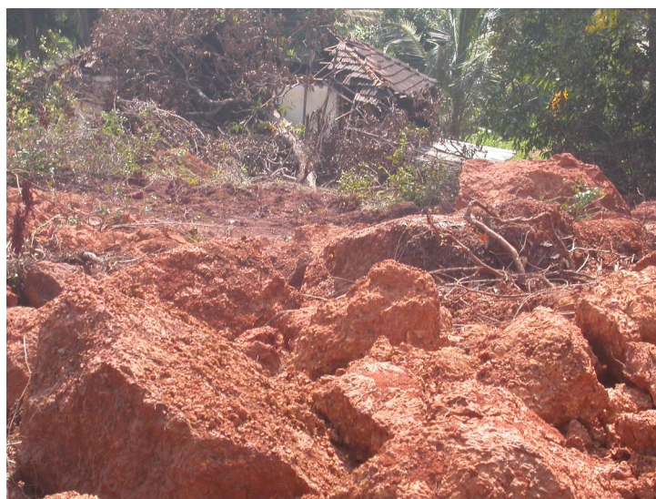
Figure 6: Incompletely formed laterite due to water logging in Kadwad-2 landslide
