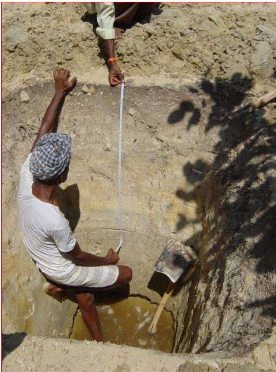
Pitting & logging of Placer Mineral Bands, Honnavar Beach Block
