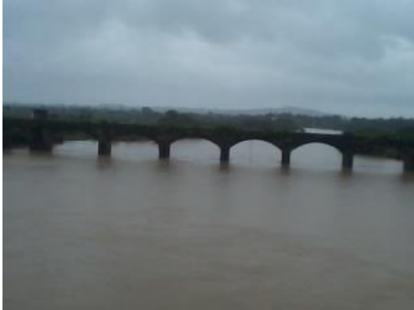
FIG -14(a) Photographic views of varada river during rainy season
