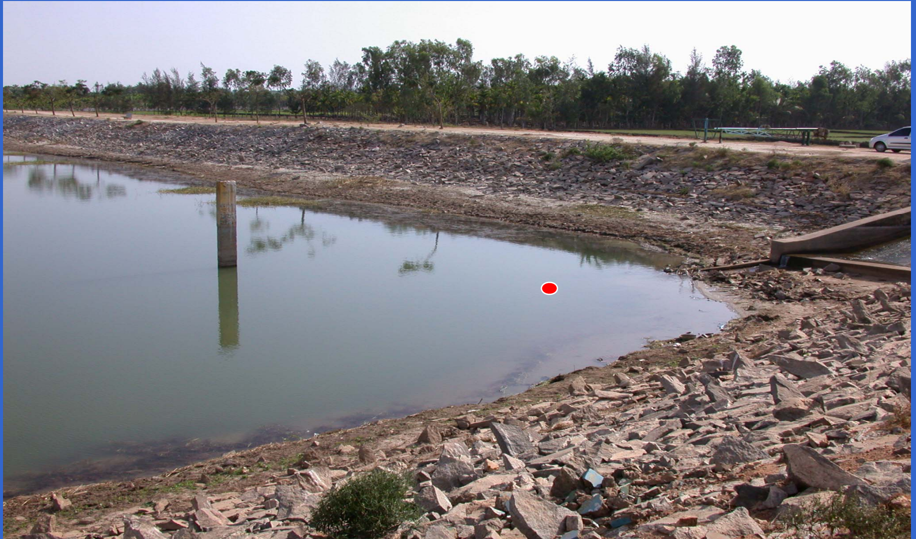
Station-1, Inlet Point
