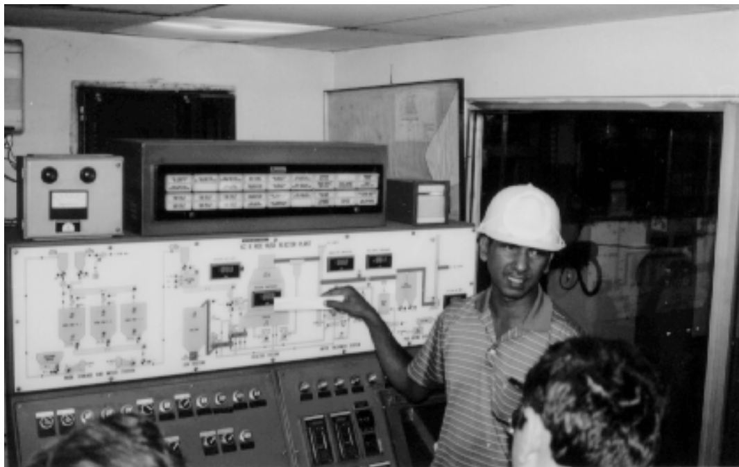
Control panel of the rice drying and packing plant
