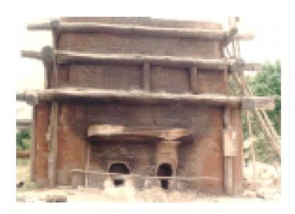
Updraft line kiln with 2 firing shafts which run over the whole width of the kiln
