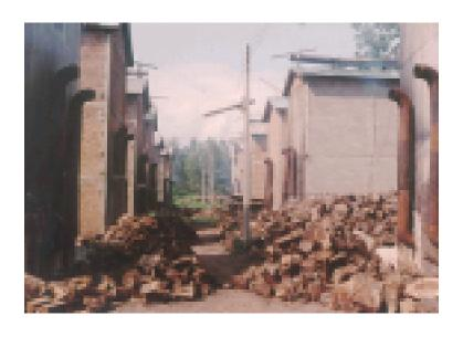
Tobacco curing barns using wood to generate process heat
