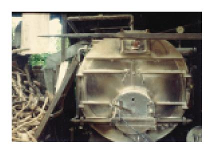
Wood/Biomass fired steam boiler used in the production of soybean sheets
