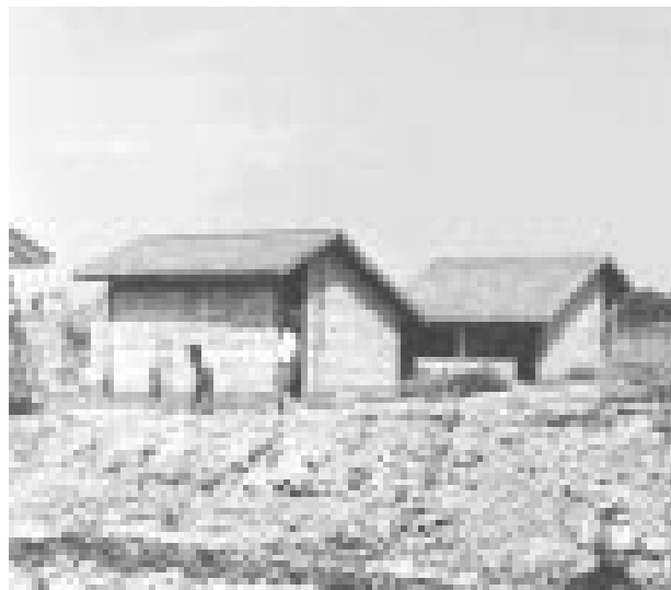
Photo 3: Peri-urban low cost housing utilizing soil/lime wall blocks.
