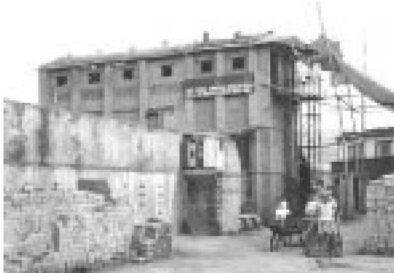
Photo 18: Chinese designed vertical shaft brick kiln in trial, Nepal.
