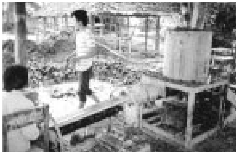
Photo 20: Brick moulding with locally made extruder.
