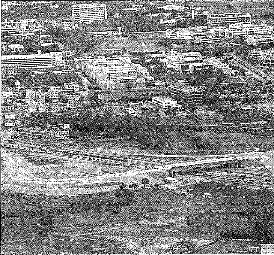
The junction where BMICP's peripheral road meets Hosur Road
