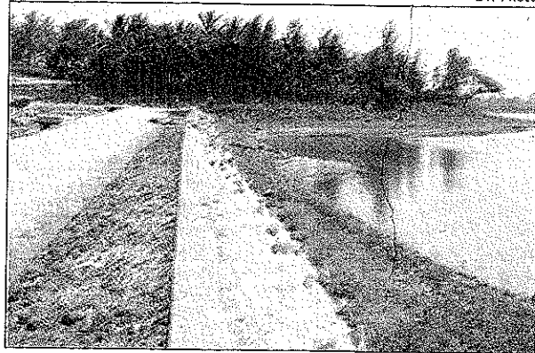
Rapid development on the banks of Hirekere lake near Nagarbhavi in Bangalore calls for concern as construction wastes are let into the lake directly.
