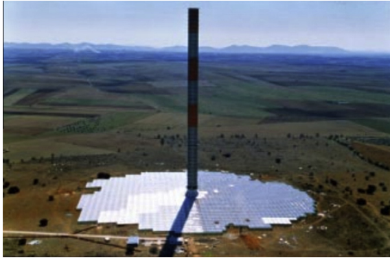
Fig. 4. Picture of Manzanares pilot plant prototype (Schlaich, 1995).
