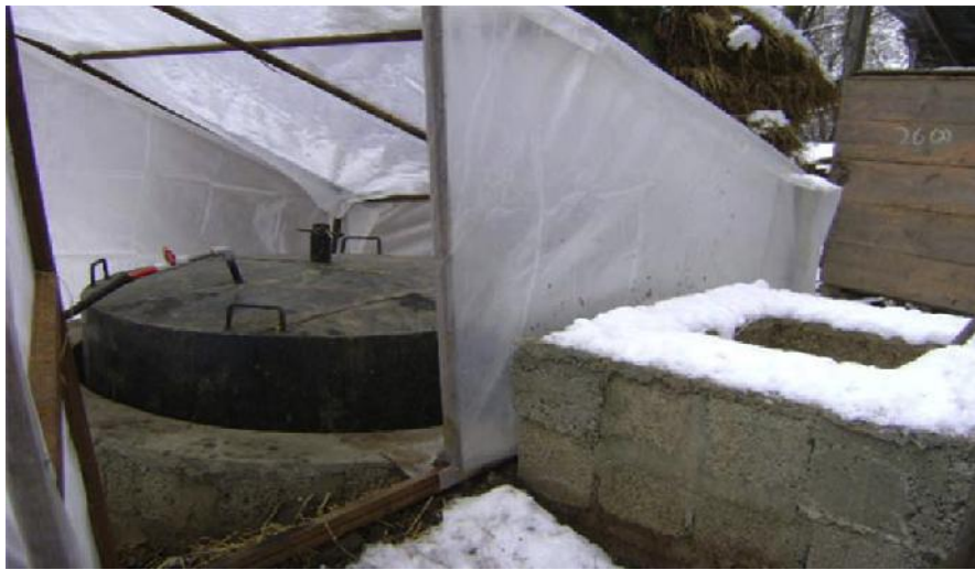
Fig. 7. The Floating drum type Biogas plant at vill. Athena Distt. Budgam.
