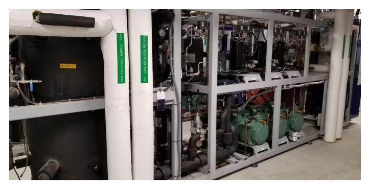
A typical grocery store refrigeration system contains large quantities of refrigerants and kilometres of pipes, along with valves and compressors with many points of connection that could potentially leak. In this system at Longo's in Stouffville, Ont., the refrigerant is CO2 (tank at left), but in many others, it is an HFC with a very high global warming potential. (Emily Chung/CBC)
