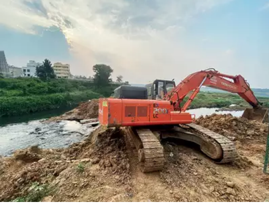
Cleaning work in progress at Bellandur Lake on Sunday
