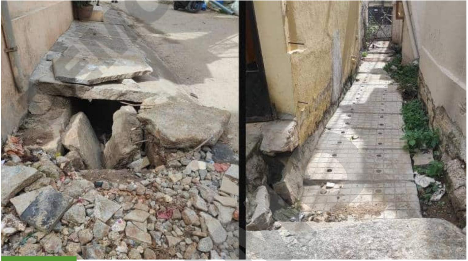
Stormwater drains in the area obstructed by debris or encroached by houses (Credit: Souptik)
