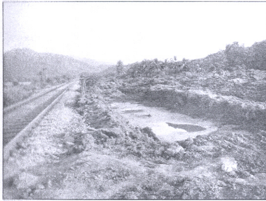
Photo10: View of the toe of the slide blocked by the embankment of Konkan railway
