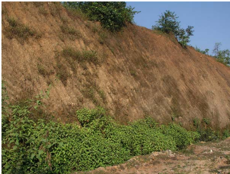
Fig: 4.4. A stable road cutting on NH-17 in Kumta showing hardened lateritic surface
