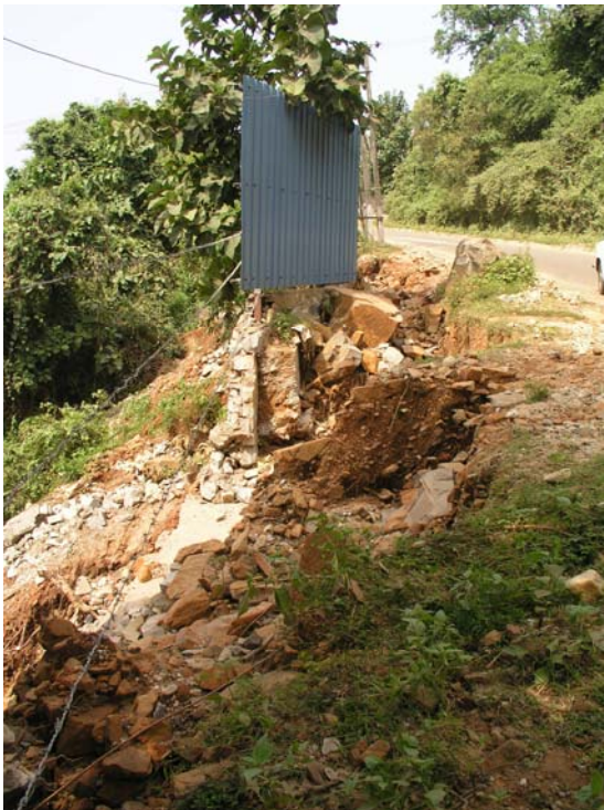
Fig. 2.7: Breach in the wall of the Naval base. Fig. 8: NH-17 cleared of debris; on the right compound wall of Naval Base
