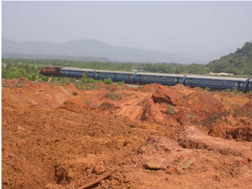
Fig. 2.16: The slide materials at Kadwad Landslide-2 stopped at the railway Embankment
