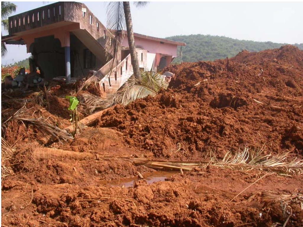
Fig. 2.14: A building that has been carried away by about 15 m in the landslide
