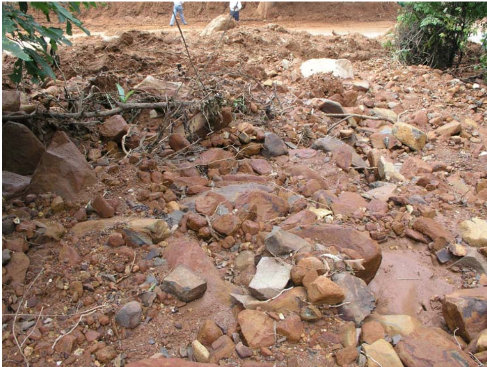
Fig 4.6: NH-17 landslide at Arga hill- unconsolidated mass of soil and granite rocks
