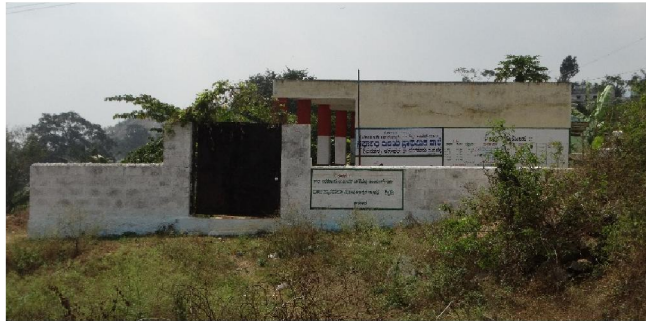
Abandoned School at Shivanahalli
