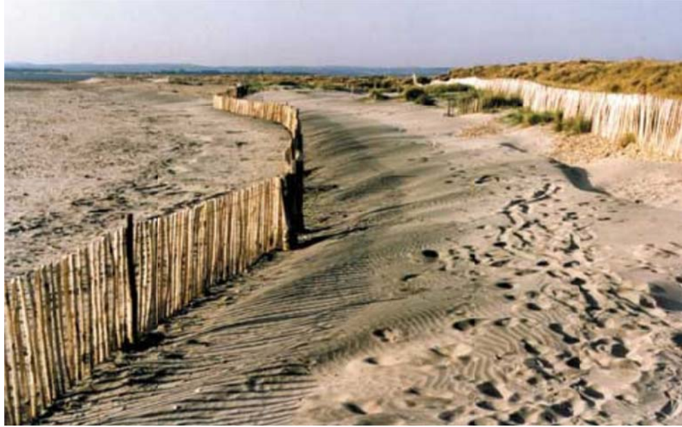
Fig. 3.6: Beach fencing parallel to the shore for development of sand dunes
