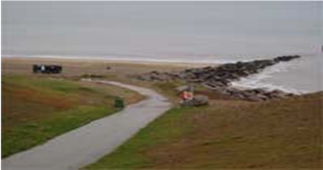
Fig. 1.6: A groyne of rocks protruding into the sea
