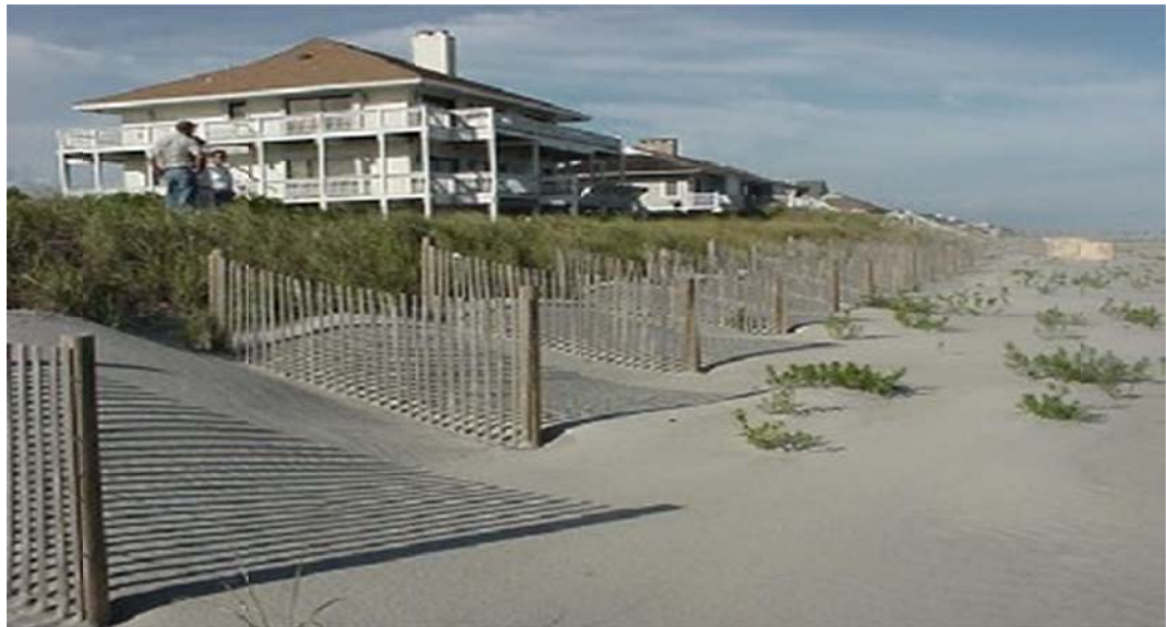
Fig. 3.5: Parallel wooden fencing vertical to the shore for sand dune development (popular in Europe)
