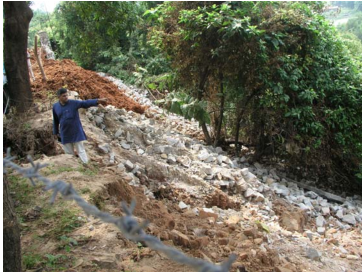
Figure 8: Landslide along NH-17, the slide material entering INS Kadamba Naval Base breaking through the compound wall
