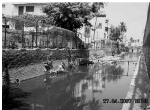
Plate 5.9: Chain link fencing to prevent solid waste dumping ( Source: BMP )
