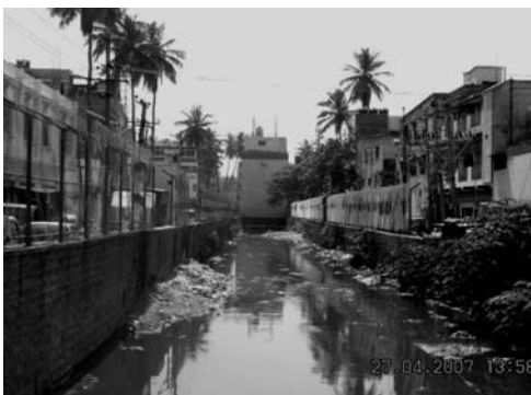
Plate 5.9: Chain link fencing to prevent solid waste dumping ( Source: BMP )
