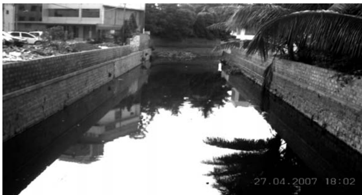
Plate 5.7: Remodelled storm water drain
