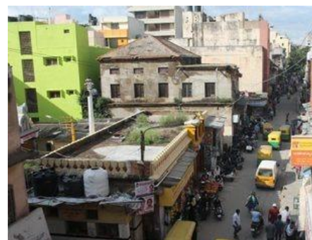
Chickpet suffers from blocked drainage systems, leaking sewerage lines and lack of public toilets.
