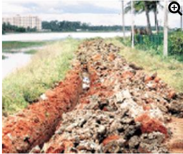
Path laying work at Jakkur Lake | EPS
