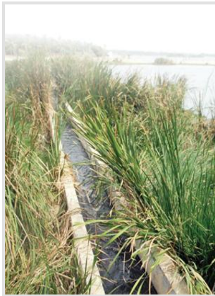
Sewage is let into the wetland for purification before reaching Jakkur Lake (in the backdrop)
